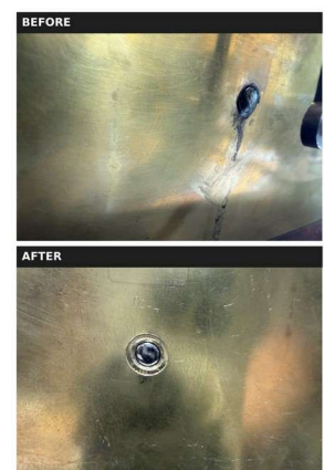
Before and after localized plate repair.
